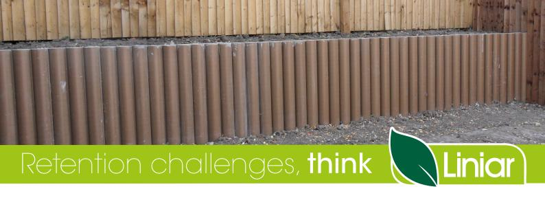
Ideal for ground stabilisation, bank retention and flood defence, Liniar's range of plastic piling offers a cost effective alternative to timber or steel – with a whole host of additional benefits for construction projects and building sites all over the UK.
